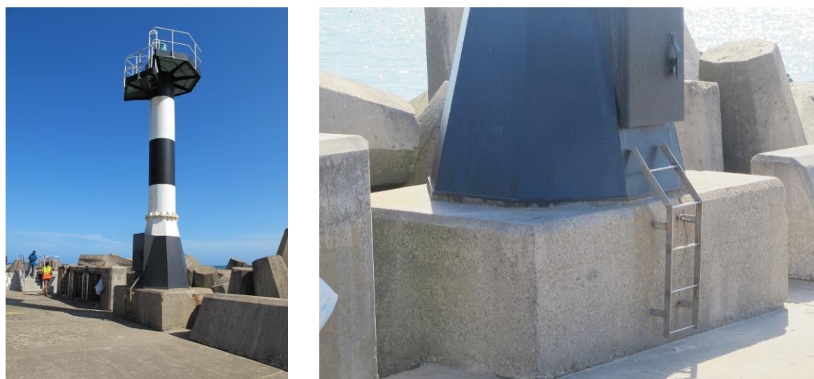
Figure 2.1.1-4: North Breakwater navigation light.
