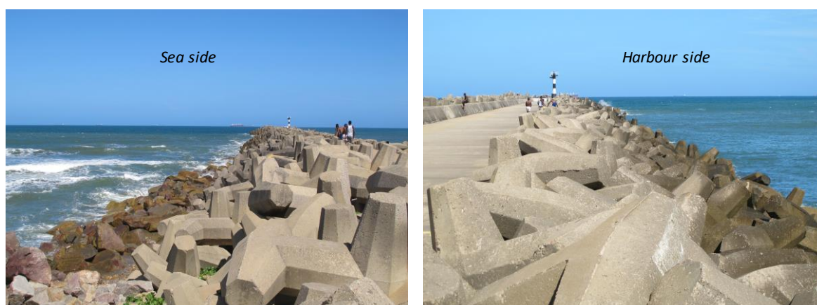
Figure 2.1.1-2: North Breakwater trunk.
