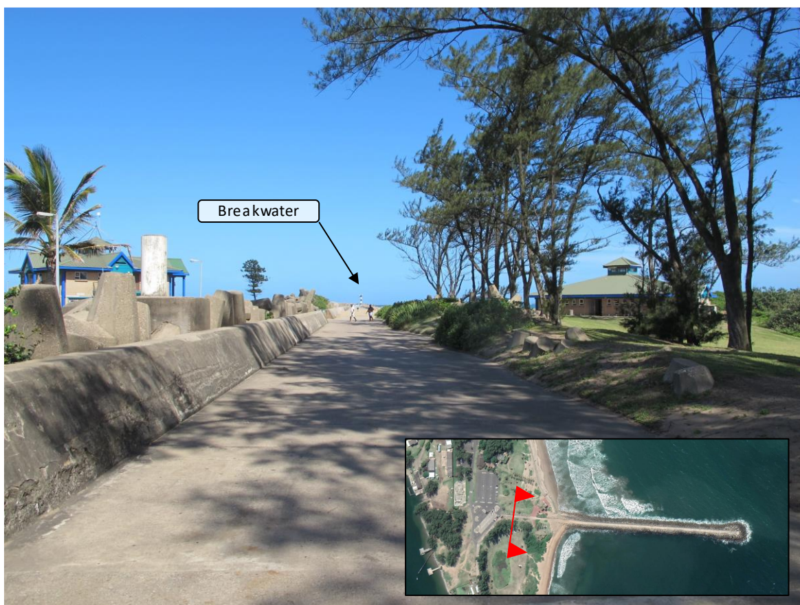
Figure 2.1.2-1: North Breakwater access.
