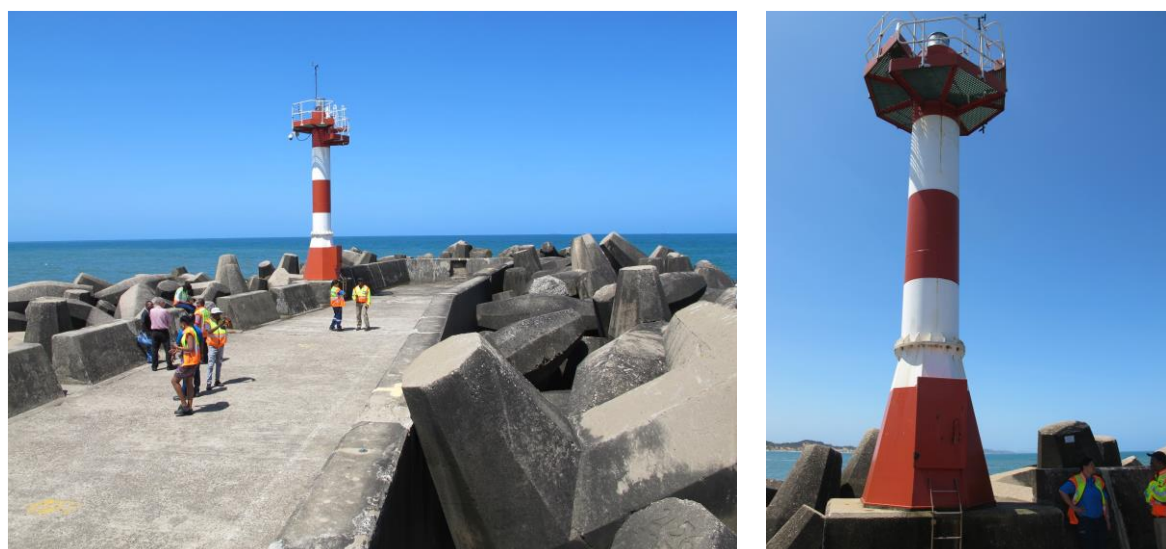
Figure 2.2.1-4: South Breakwater navigation light.
